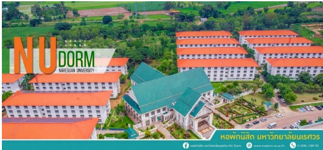
Figure 20 The surrounding of NU Dormitory
