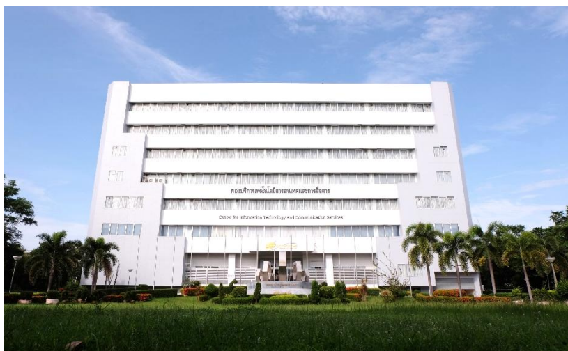
Figure 25 Center for Information Technology and Communication Services (CITCOMS) building
